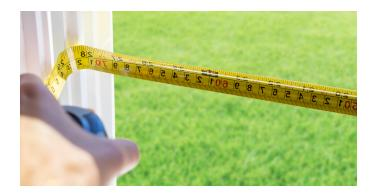
Now, measure the height, from the bottom window sill to the bottom of the top window's sash. Again, identify the two whole numbers that the measurement falls between. In the example below the range falls between 28" and 29".
